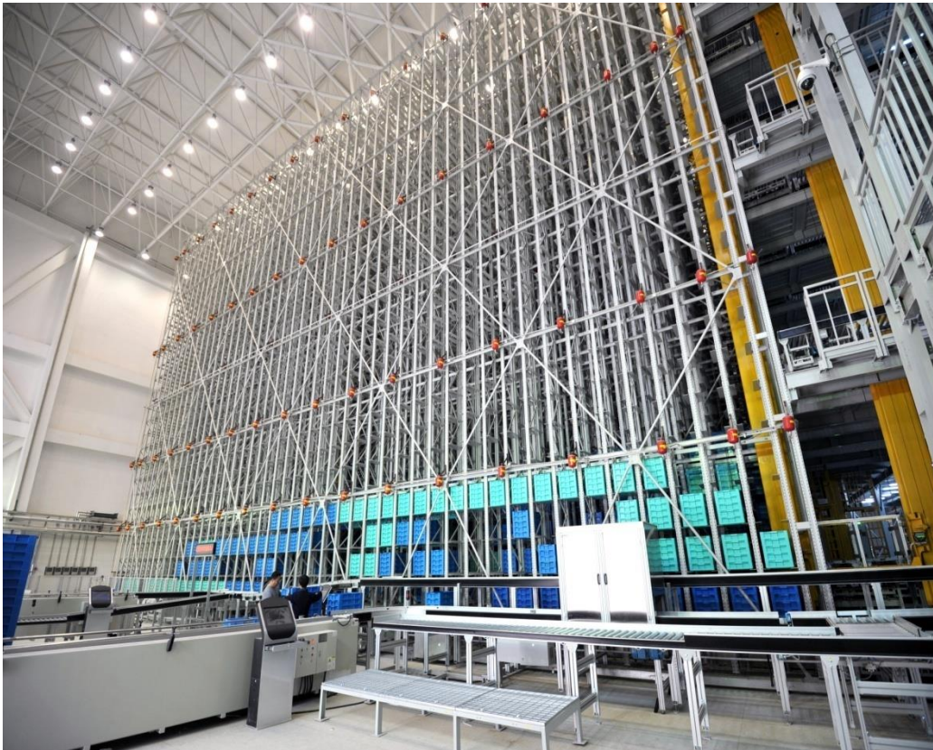
AS/RS (Automatic Storage and Retrieval System)
