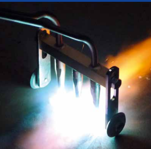
Flame Straightening Flame Straightening
